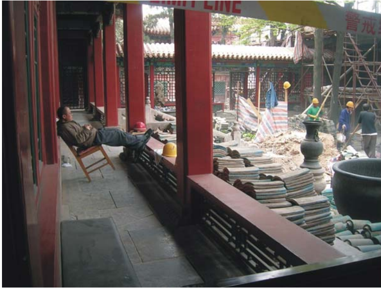
Restoration of Buildings in the Forbidden City
